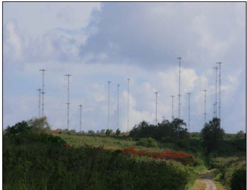
Figure 12.1-4. Antenna Array of Mariana Relay Station
